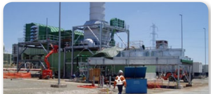
Gas turbine generator unit - during installation in SA
