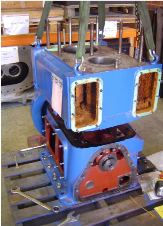
Disassembly of Compressor for Inspection
